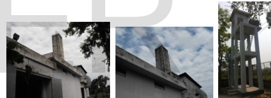
Fig 3.1b: Lighting system around the CWPSF and watch tower
