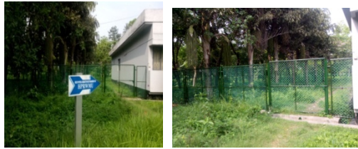
Fig 3.2.a: 2 meter high nuisance fence along the site boundary parallel to the CWPSF and SSDL
