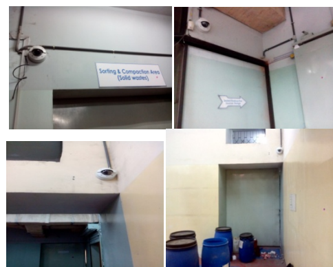
Fig 3.1c: 4 Surveillance cameras 3.2 Delay Systems at the Central Radioactive Waste Processing and Storage Facility (CWPSF)
